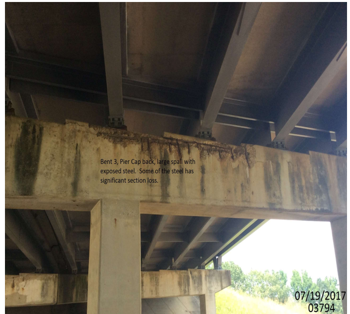
PHOTO 2 Description Spall @ Bt. 3 cap, back.
