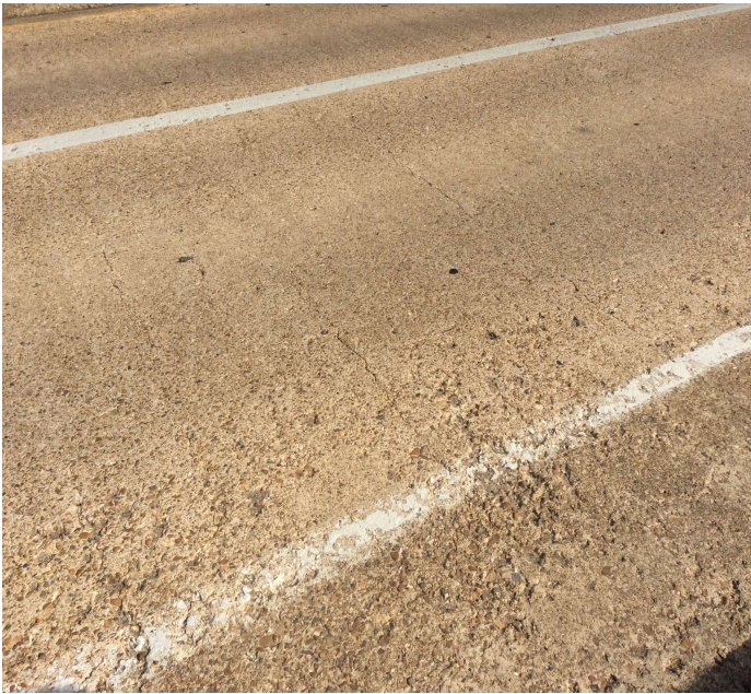
PHOTO 1 Description 03794 deck cracks span 1 rt.
