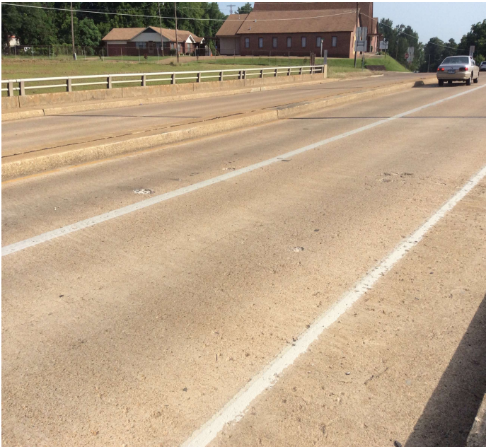
PHOTO 4 Description 03794 span 2 right deck cracks and potholes.
