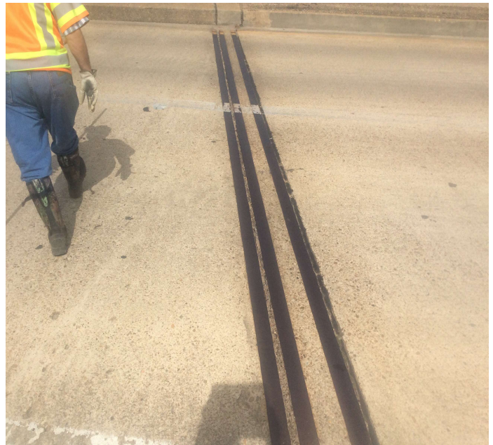
PHOTO 2 Description Joint at abutment 2, this is typical of all joints.
