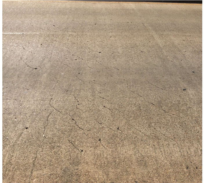
PHOTO 5 Description 03794 span 4 lt. Cracks
