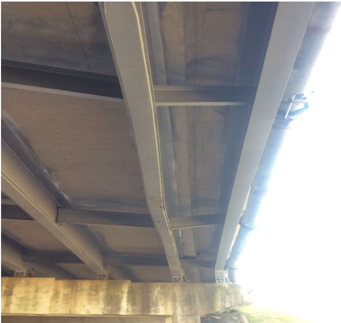
PHOTO 1 Description 03794 Girder 2 span 2 showing bending from traffic impact.
