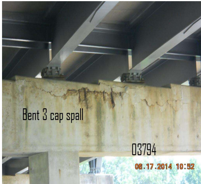
PHOTO 1 Description 2014 inspection photo. 03794 Bt 3 cap spalls with exposed steel.
