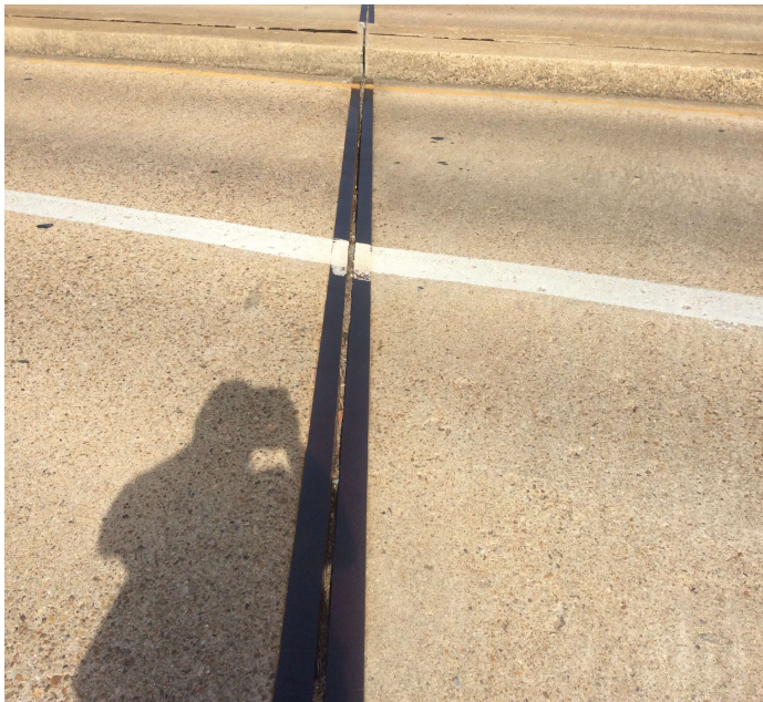
PHOTO 1 Description 03794 joint material @ Bt 2 joint.
